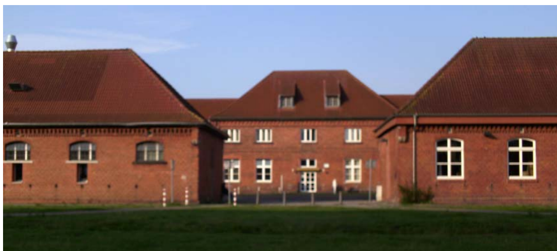
Archives Building, Muenster University
