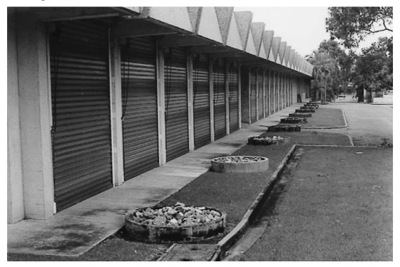
The National Archives of Australia uses circular rock pits at its Darwin facility to drain water away from the building. Water falls from the roof into the pits and is drained away via underground channels.
